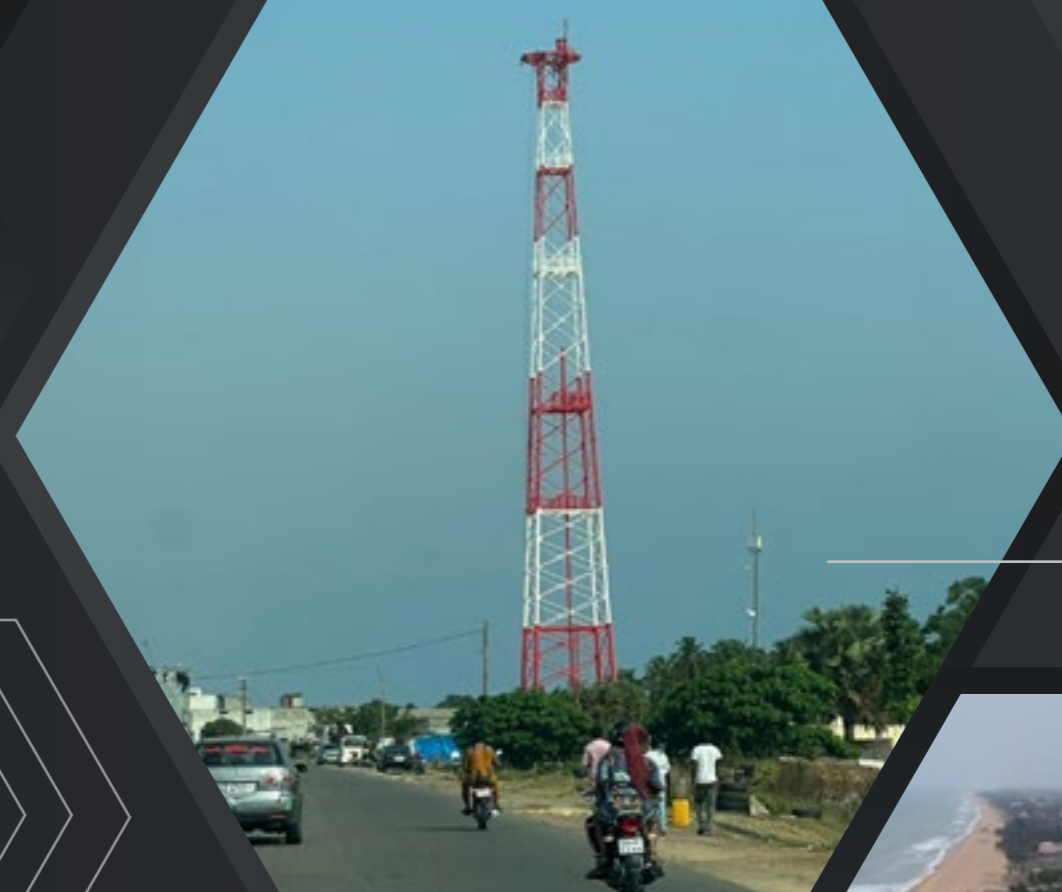
TELECOMMUNICATION TOWER BENIN
