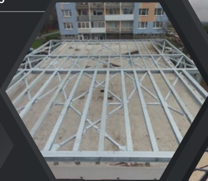
PHOTOVOLTAICS STRUCTURE FOR TEHO KOŠICE
